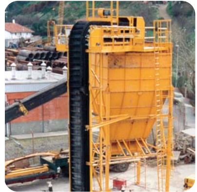
Civil work | Chile
